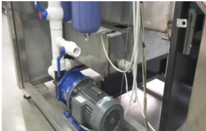
Plumbing and Pumping Systems
